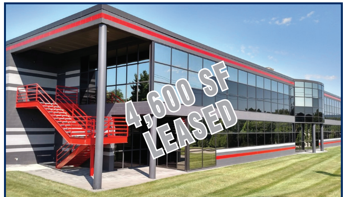
4201 Crums Mill Road, Harrisburg, PA
